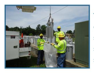
Transformer Bag Kits are an easy, cost effective way to transport and store leaking transformers. Different sized kits are offered to cover all sized transformers
